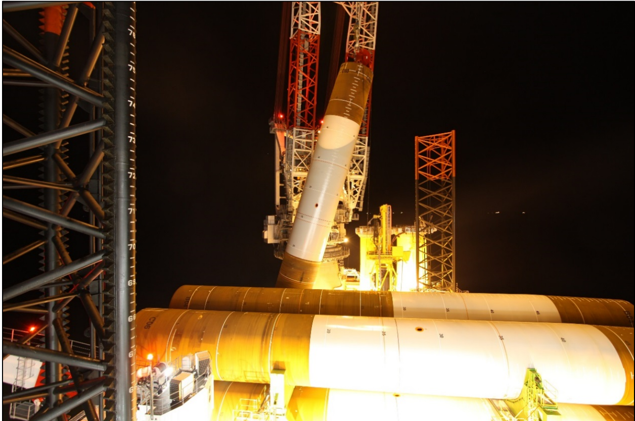
Figure 10.2 Transportation and Installation of a Monopile (Westermost Rough, 2014)
