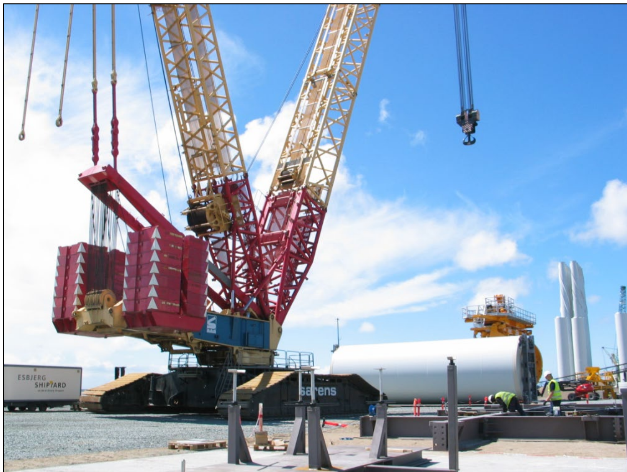
Figure 10.4 Upending of Tower Section in Load Out Port (Gode Wind, 2015)
