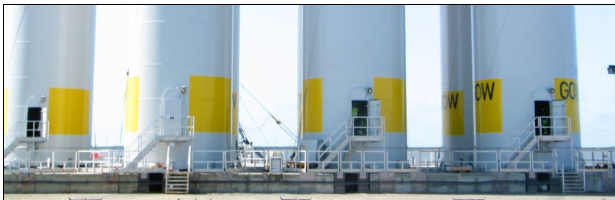
Figure 10.5 Towers Assembled and Ready at the Load Out Port (Gode Wind, 2015)
