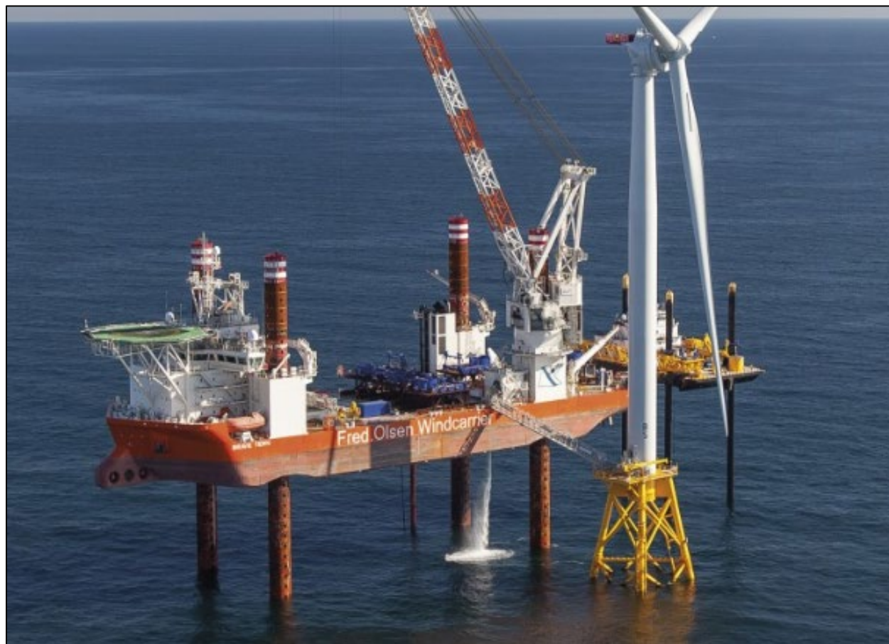
Figure 10.10 WTG Installation Vessel and feeder jack-up barge at Work - Installation of a WTG Blade (Block Island, 2016)
